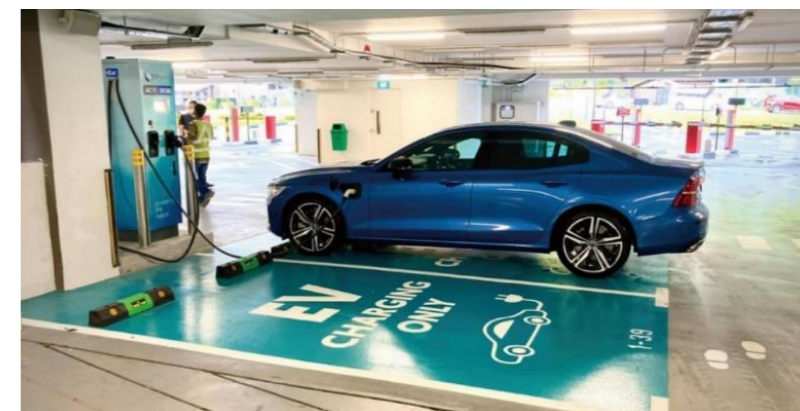
EV Charger Installation in Singapore
